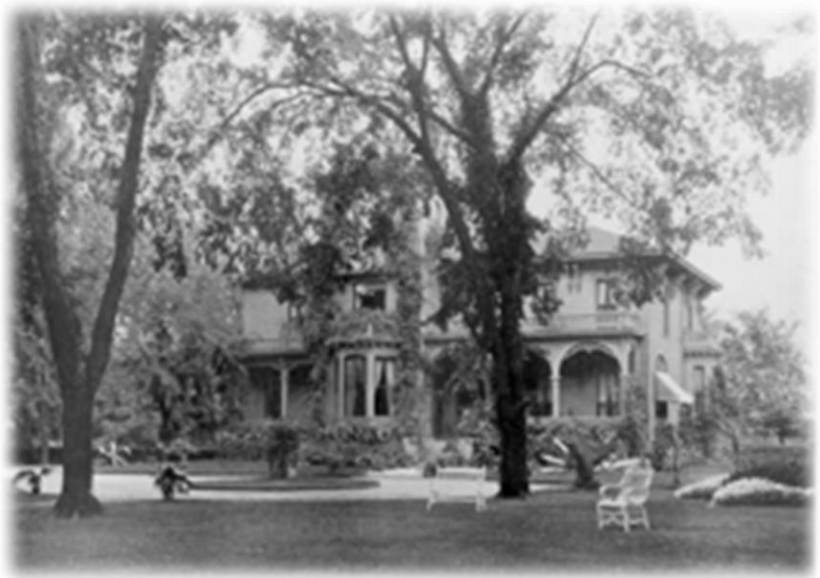
Figure 2: Villa Rosa, Dorilus' home at the current site of Mia. Courtesy Hennepin County Library.
