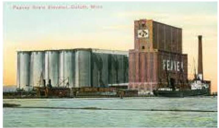
Figure 4. Peavey grain elevator built in 1900 still in operation today http://www.allposters.com/-sp/Peavey-
