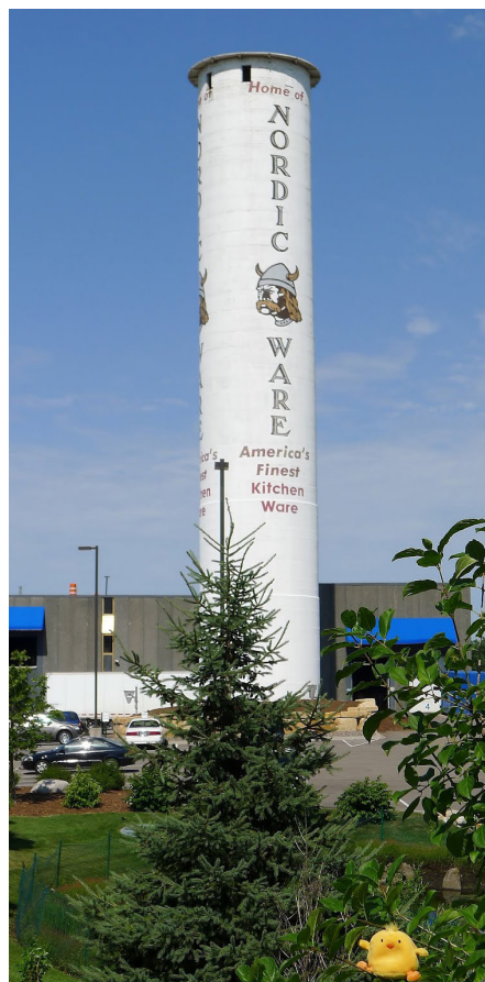
Figure 3. The Peavey-Haglin Experimental Concrete Grain Elevator built 1899-1900
